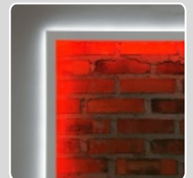
frame mounted around a wall niche; first LED strip - red, the other cool white
